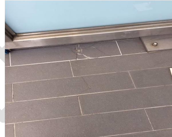
Cracked tiles on balcony
