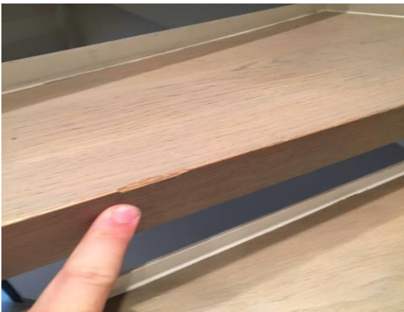
Chipping to stair edges
