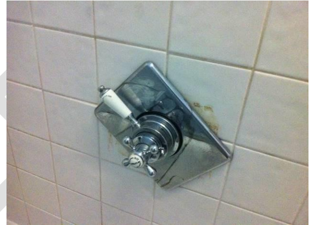
3. Bathroom shower tap back plate loose.
