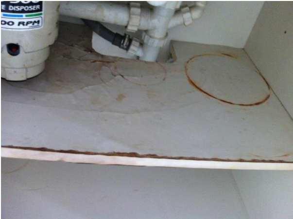
4. Staining & cracking to sink cupboard laminate.
