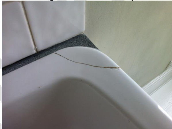
5. Crack to kitchen sink.
