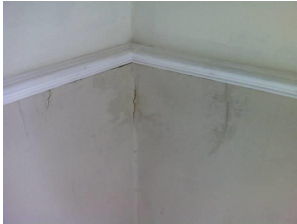
8. Damp staining to reception wall.
