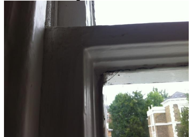
6. Crack to reception window.
