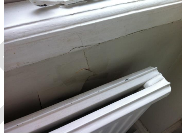
3. Stress cracking to kitchen wall.
